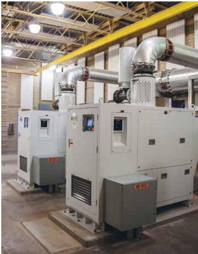
New 200-horsepower turbo blowers that adjust power consumption during the aeration process were installed at the Southeast Wastewater Treatment Plant.
